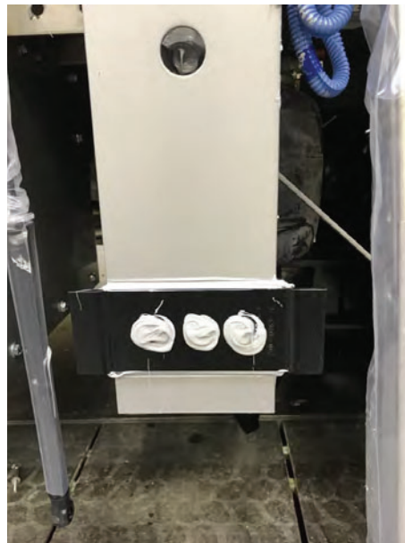
Sealed & powder coated aluminum skirt panel bracket
